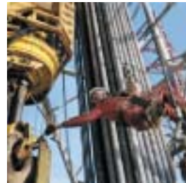
Above the drilling rig floor, offshore Vietnam
